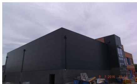
Cladding to the sports hall is complete.
