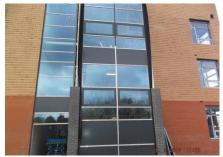
The curtain walling to the east elevation staircase is installed.
