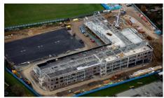
The construction of the structural steel was completed in early December 2015 followed by the concrete slabs just before Christmas in all zones. The SFS framework with insulation is also complete and the brickwork package is progressing well (see photo 1).
